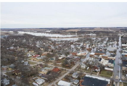
Flood damage in Hamburg, Iowa.
